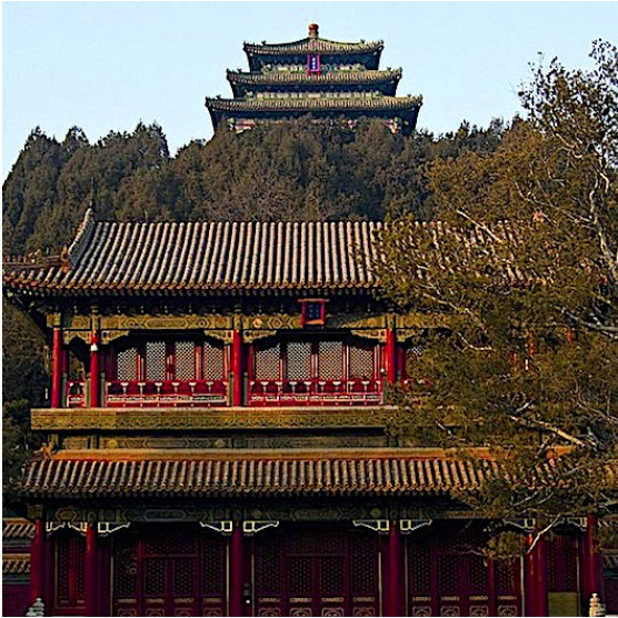
Figure 28a: A recent photograph of Prospect Hill. Source: Wikimedia Commons
